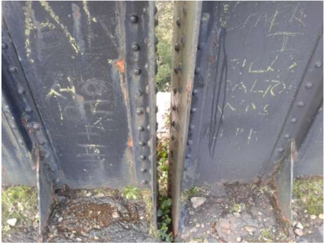
Figure 7 : View of expansion joint.
