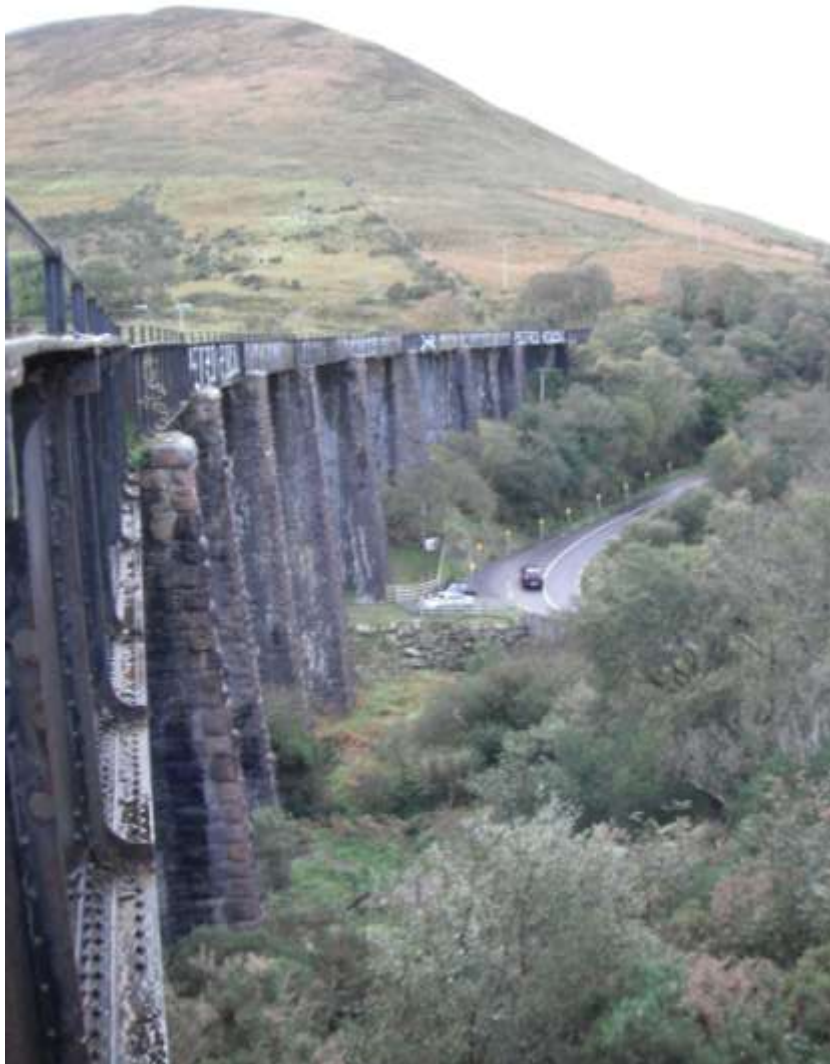
Figure 1 : General view along bridge from the east.
